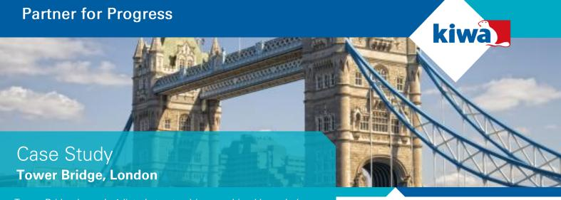
Tower Bridge (a grade 1 listed structure) is a combined bascule (a moveable bridge with a counterweight) and suspension bridge built between 1886 and 1894. The bridge crosses the River Thames close to the Tower of London and has become an iconic symbol of London.
